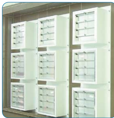
Intake side of a 3x3 FANWALL array showing the backdraft dampers to isolate the fans when turned off.
